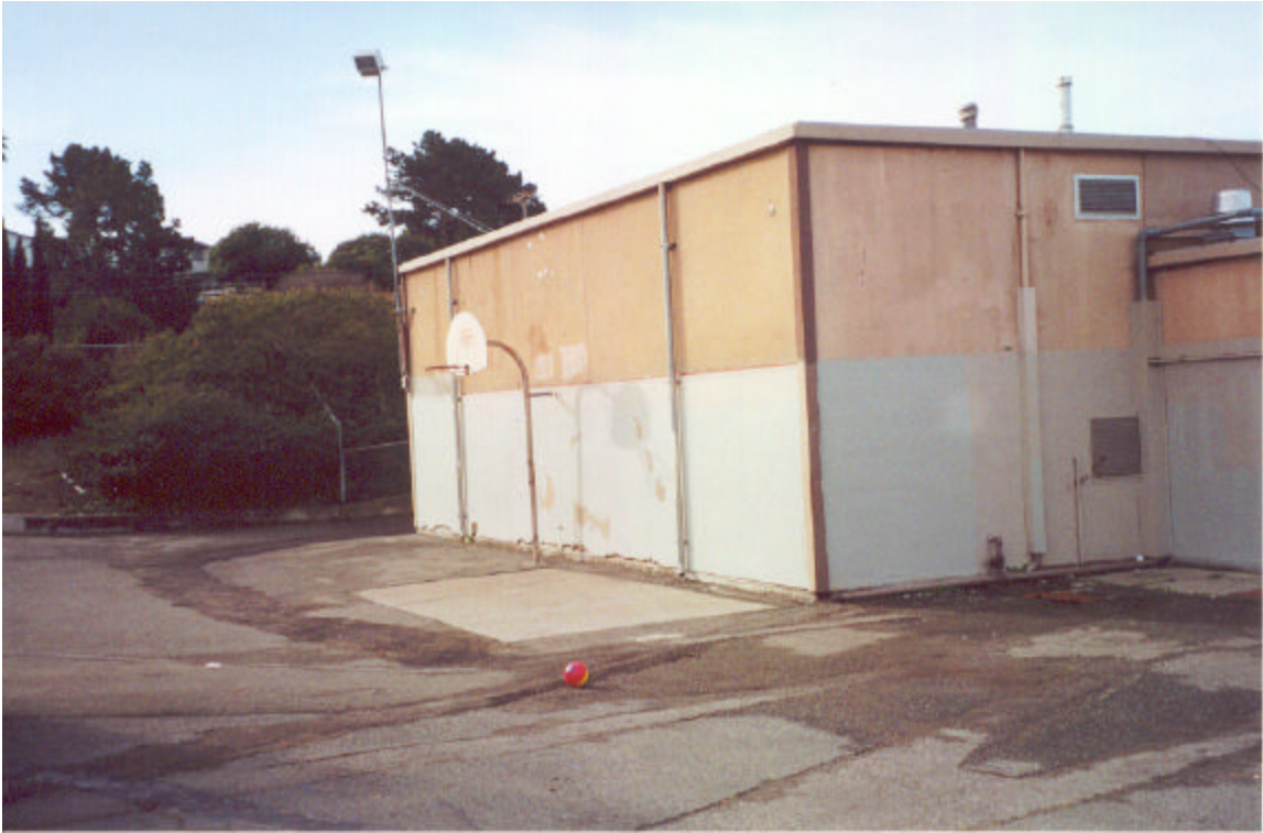
Figure 4: East Face of Multi-Purpose Building
