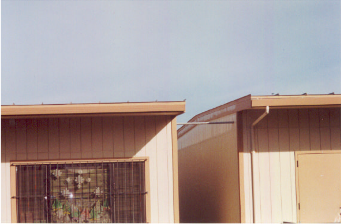
Figure 14: Conduit Running between Portable Classrooms
