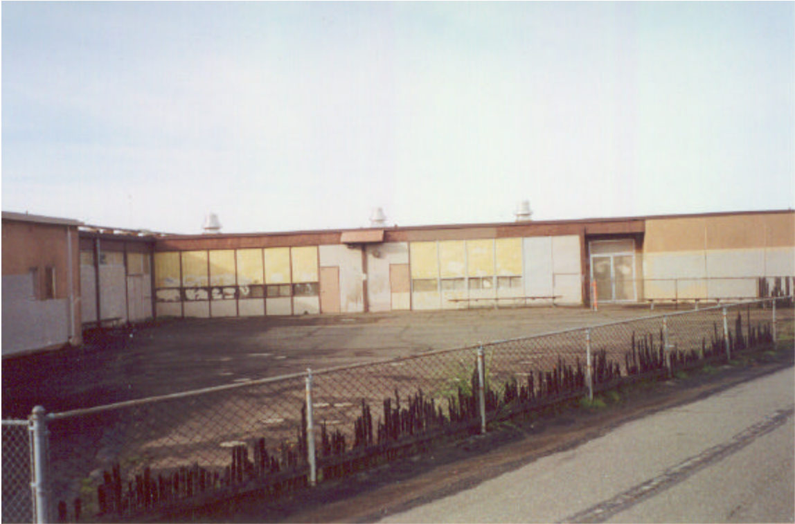
Figure 6: East Face of Main Building
