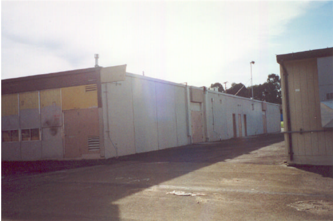
Figure 8: West Face of Main Building
