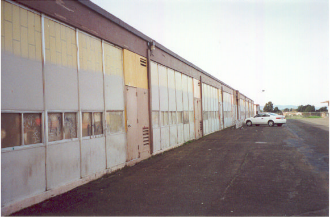
Figure 7: North Longitudinal Wall of Main Building
