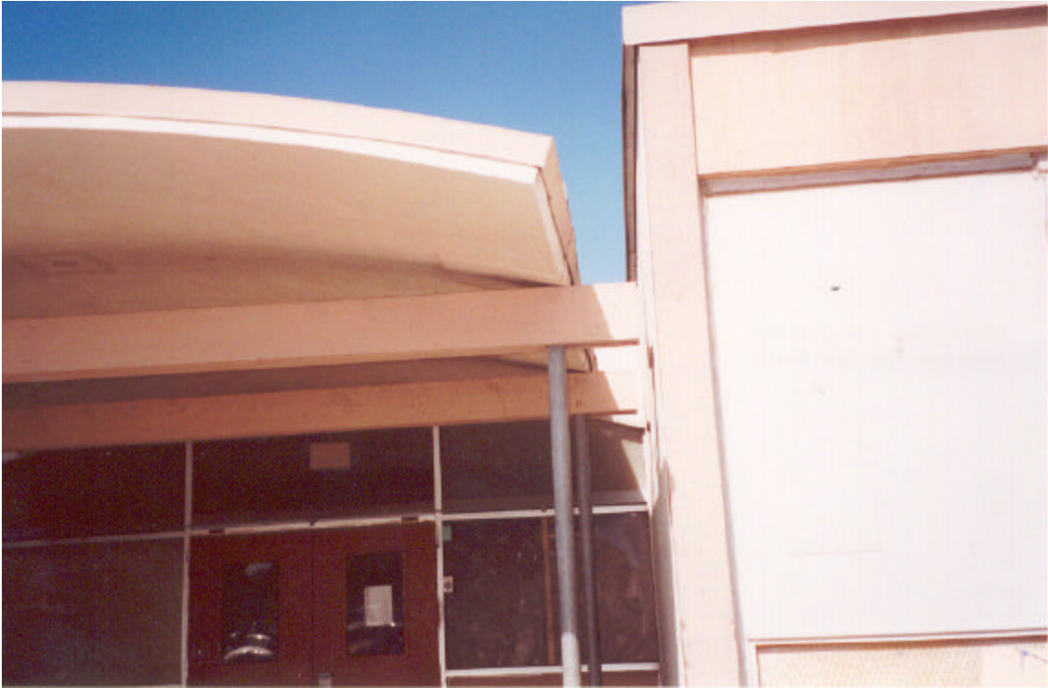
Figure 15: Entrance Canopy at Main Building
