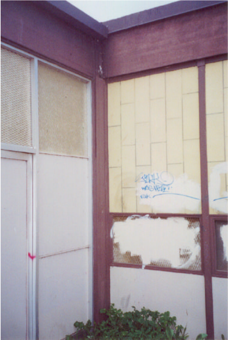
Figure 16: Seismic Joint at Corridor near Main Building
