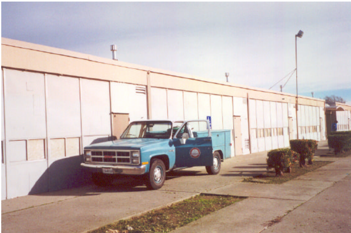
Figure 9: South Longitudinal Wall of Main Building (West Half)
