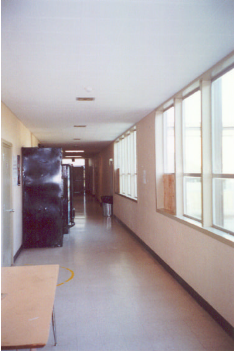
Figure 10: Interior Corridor of Main Building at Courtyard Windows
